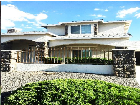
ARIZONA WATER DAMAGE
