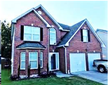
GEORGIA TONATO DAMAGE
