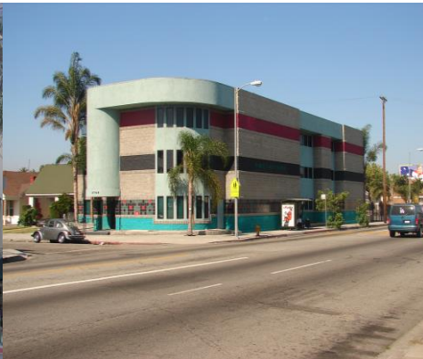
CALIFORNIA WATER DAMAGE
