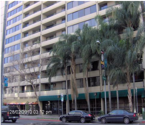
CALIFORNIA WATER DAMAGE
