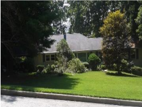
NORTH CAROLINA WATER DAMAGE
