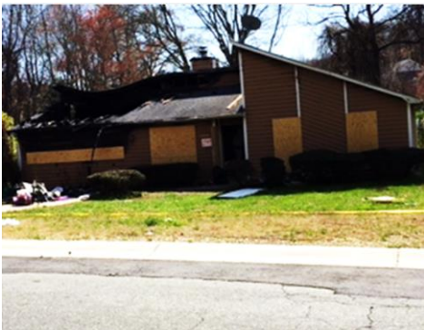
NORTH CAROLINA WATER DAMAGE
