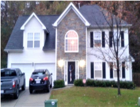
NORTH CAROLINA WATER DAMAGE
