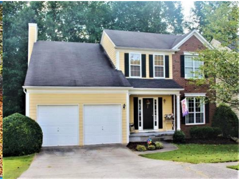
GEORGIA WATER DAMAGE
