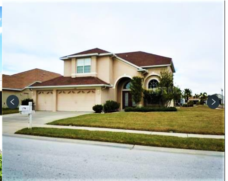
FLORIDA WATER DAMAGE
